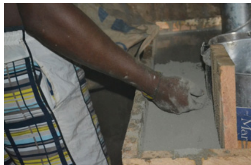
66 Agregando cemento gris
